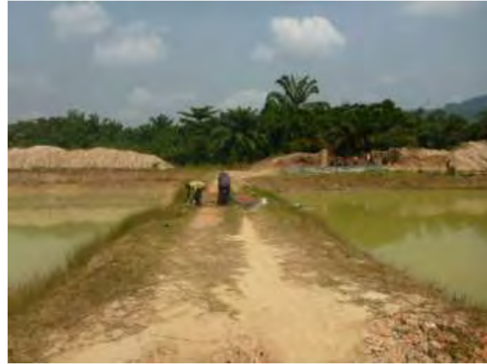
FIGURE 5 - CLAY-RICH SOIL BORROW PLOT
