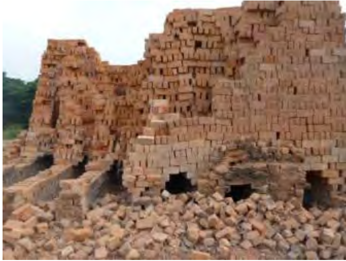
FIGURE 10 - PARTIALLY DECONSTRUCTED CLAMP KILN
