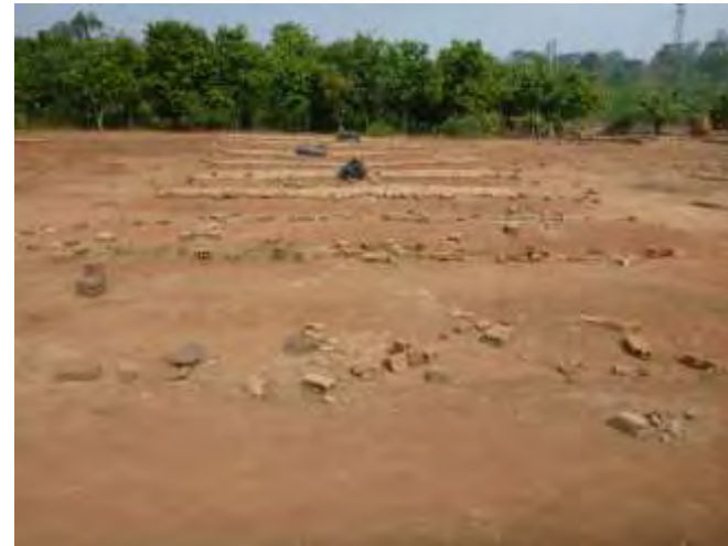
FIGURE 16 - DRYING GREEN BRICKS IN OPEN AIR
